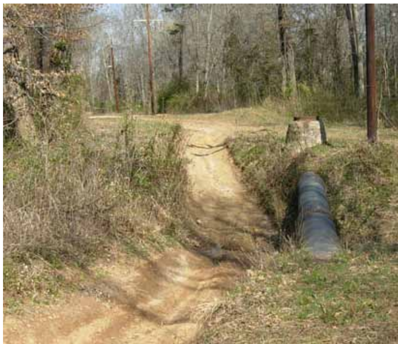
Photo 1 - Sewer Line Trail along Abbotts Creek near US 64
