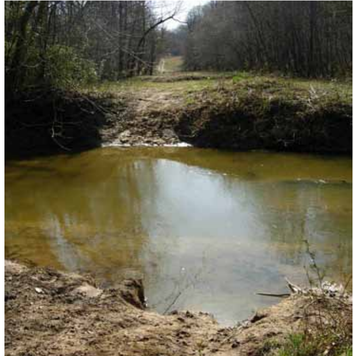
Photo 3.3 – Abbott's Creek at Natural Gas Pipeline Crossing South of Lake Thom-A-Lex Dam
