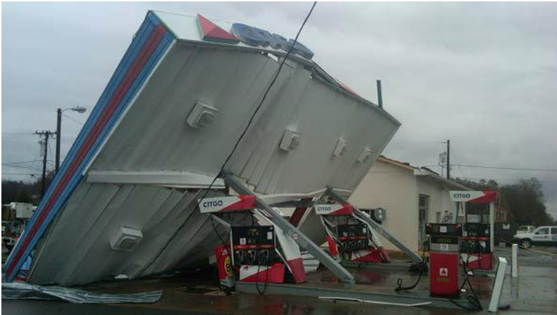
Tornado damage (11/2011), Davidson County, NC Photo Source: ABC11.com
