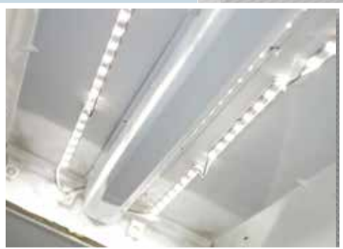
Old fluorescent lighting above. New LED lighting, below.
